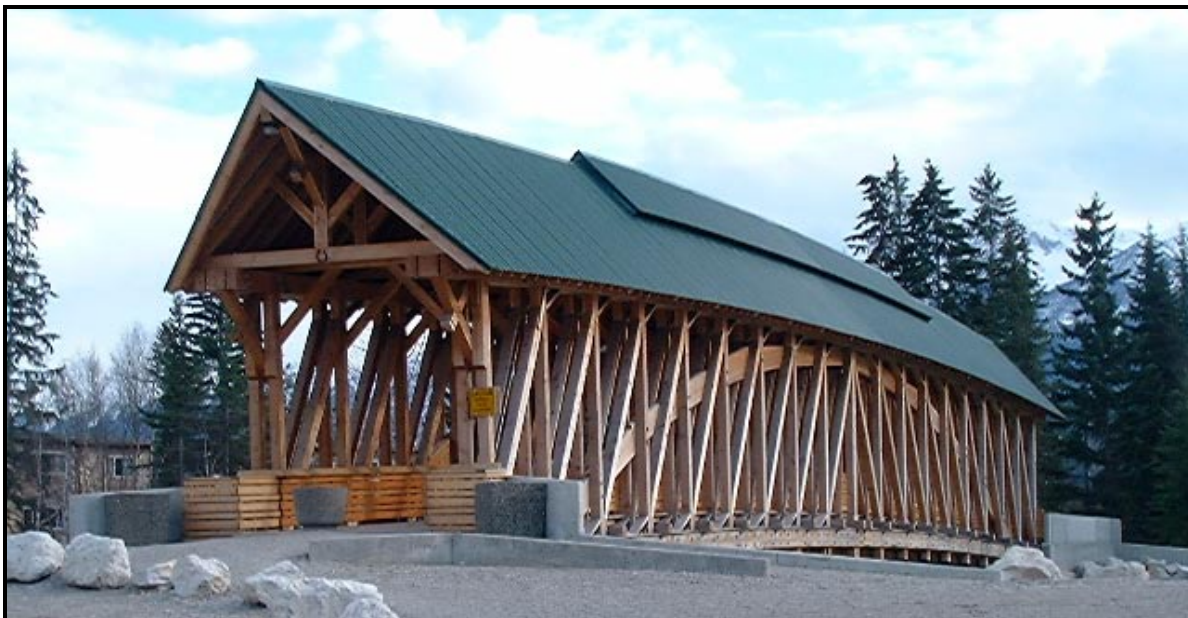
Figure 10: Timber frame walking bridge across the Kicking Horse River in Golden, BC. The logs were donated by Members of the Columbia Woodlot Association.
