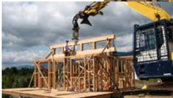
Russel McBride helping build school house May 2009
